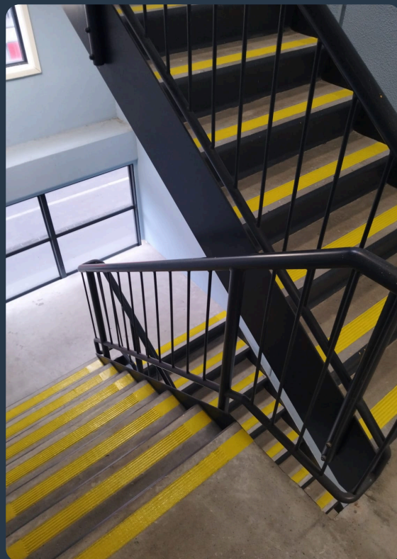
Traffic Yellow treads, top to bottom of a commercial stairwell.
