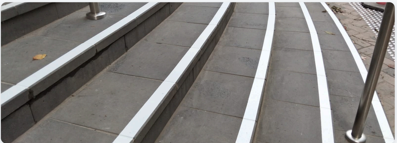
White stair nosings rolled straight onto curved bluestone steps. No strips, no drilling.
