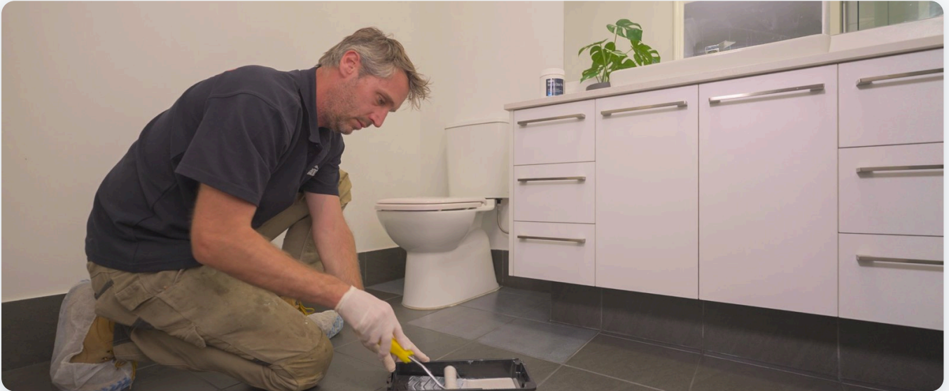
A certified installer laying down Stellmann Non-Slip Clear in a residential bathroom. Clean, prime, one coat, done.
