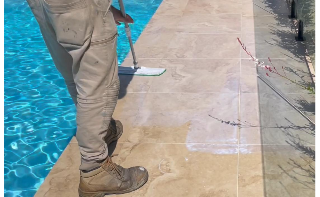
Primer application to travertine tiles
