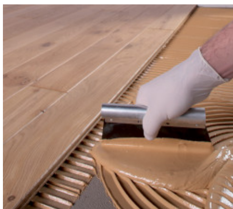
Application of Ultrabond P990 1K
