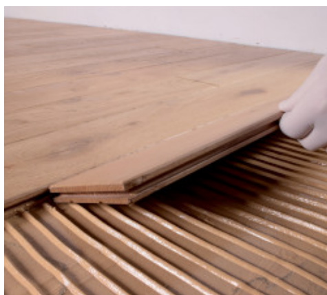
Installing wood flooring
