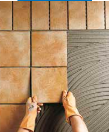
External installation of klinker tiles
