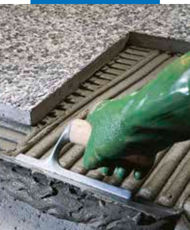
External installation of relief terrazzo "graniglie" tiles
