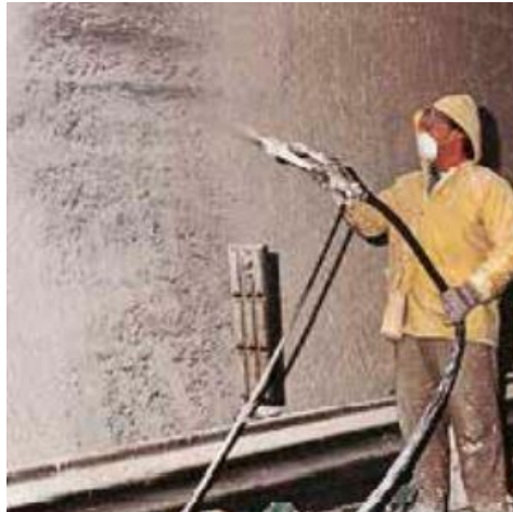
Application of Planiseal 88 by spray gun in highway tunnel
