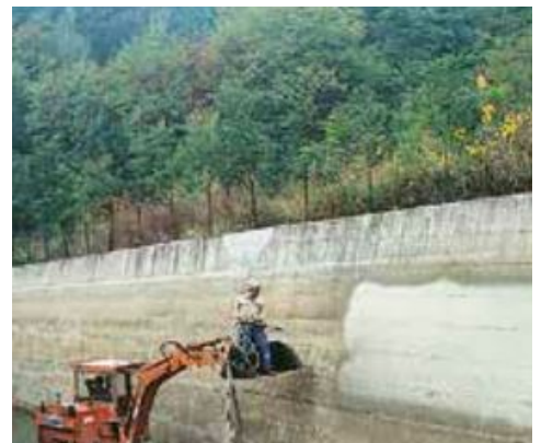
Application of Planiseal 88 by spray gun in hydroelectric canal
