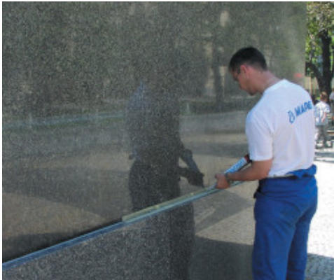
Sealing a façade joint with Mapesil LM
