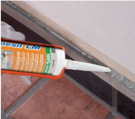
Sealing a fillet joint on natural stone
