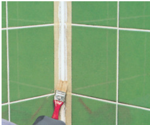
Smoothing the joint with soapy water and a small brush
