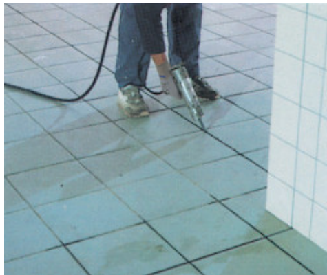
Sealing ceramic tile floor with Mapesil AC
