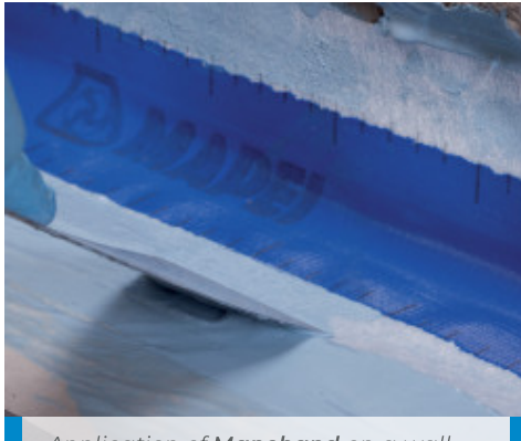
Application of Mapeband on a wall-floor fillet joint with Mapelastic AquaDefense
