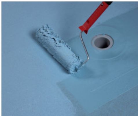
Application by roller of the second coat of Mapelastic AquaDefense
