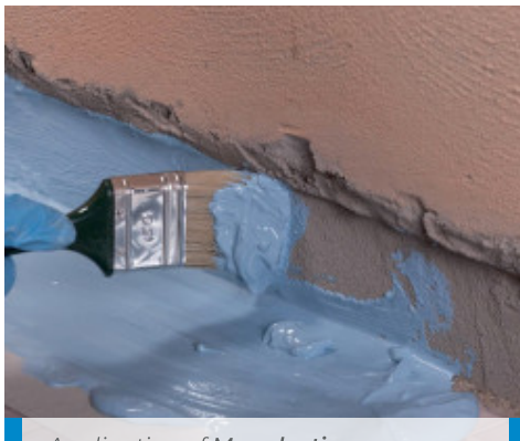
Application of Mapelastic AquaDefense by brush between floor and wall before applying Mapeband
