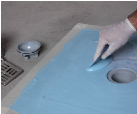
Impregnating Drain Vertical fabric with Mapelastic AquaDefense
