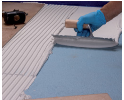
Bonding tiles on Mapelastic AquaDefense
