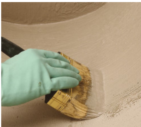
Waterproofing of details by brush
