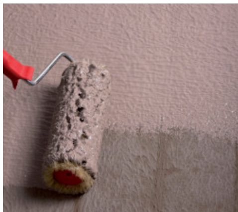
Waterproofing of details by roller
