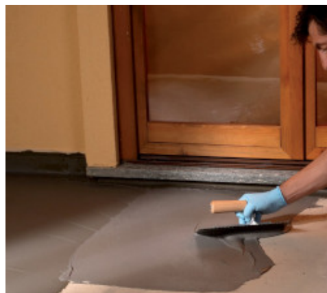
Waterproofing of terraces by trowel
