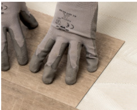
Installation of LVT with Ultrabond Eco V4 Evolution
