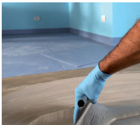
Applying Ultrabond Eco 380
