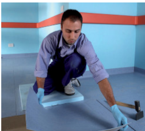
Installing PVC floor tiles
