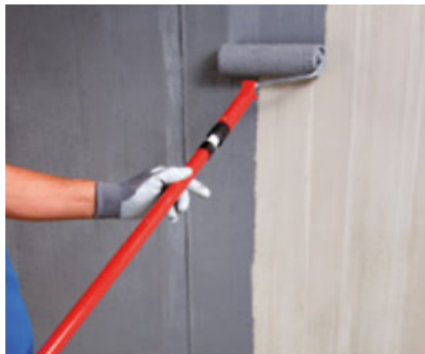
Application of Eco Prim Grip on concrete by roller
